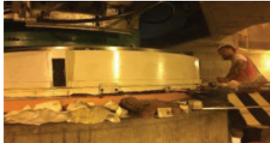
LEFT: Spokane St Swing Bridge: Pier 6 lift cylinder emergency replacement June 2018
