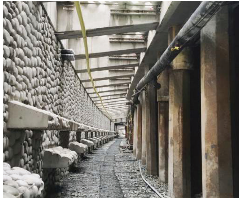
Elliott Bay Seawall
