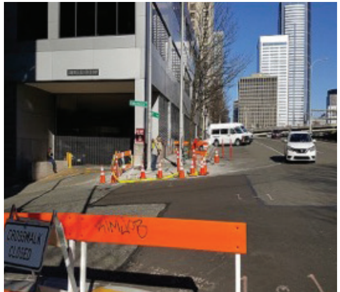
RIGHT: Sidewalk reconstruction at 6th Ave and Columbia Street
