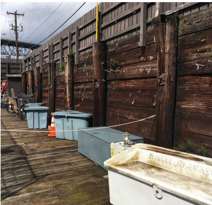
N Northlake Way Retaining Wall
