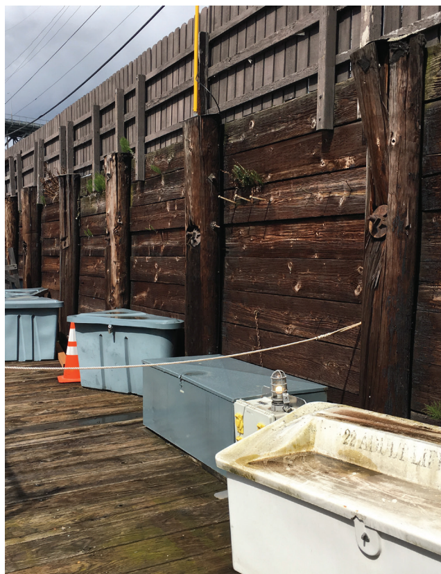
Northlake retaining wall
