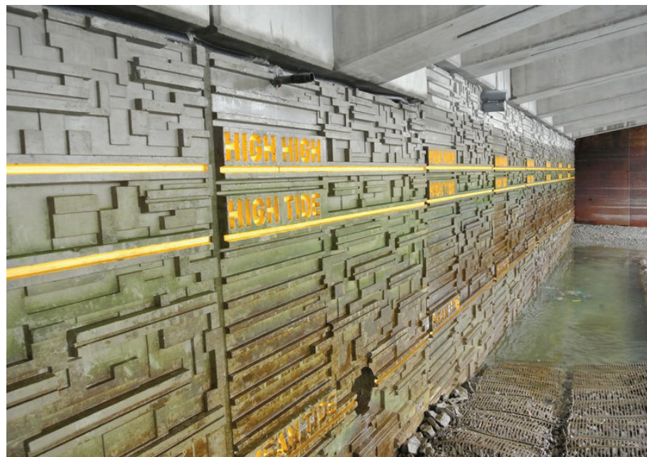
Seawall Tide Line Markers
