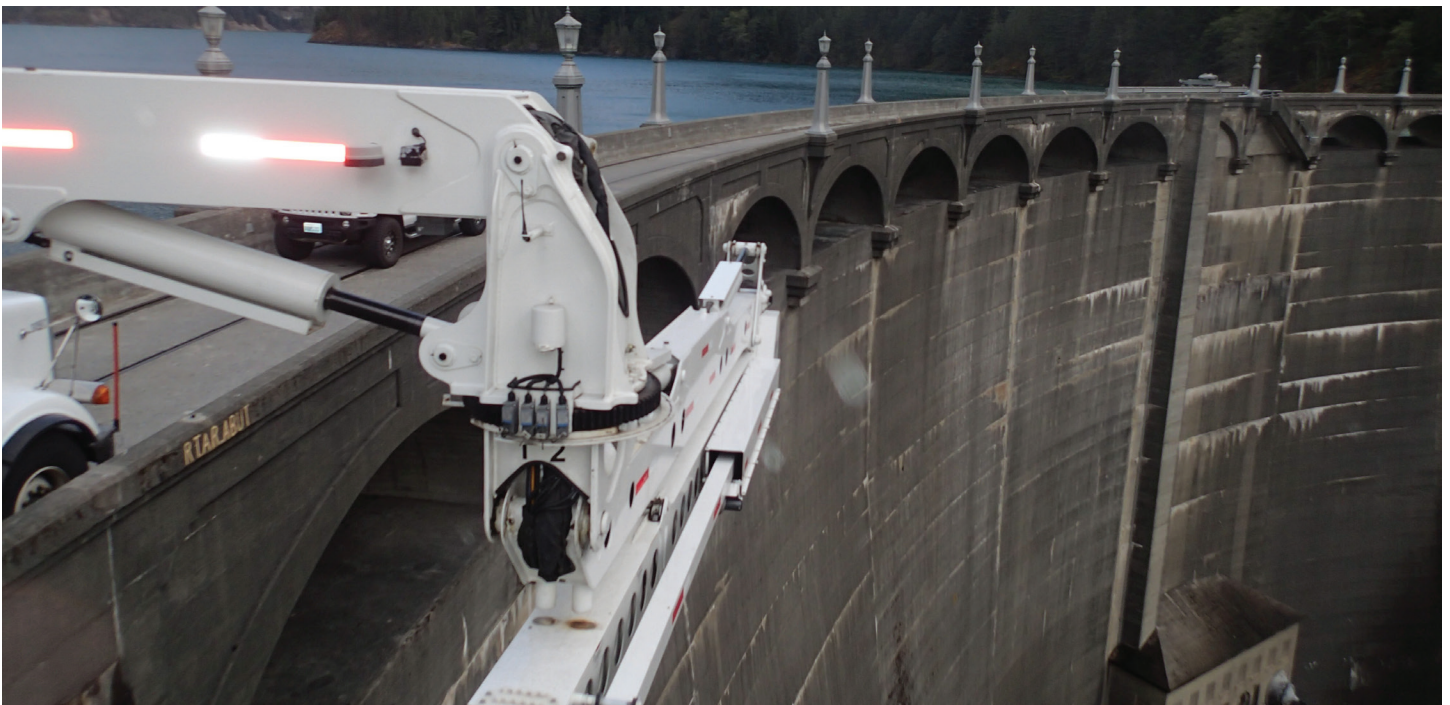
Light Diablo Dam Bridge Inspection
