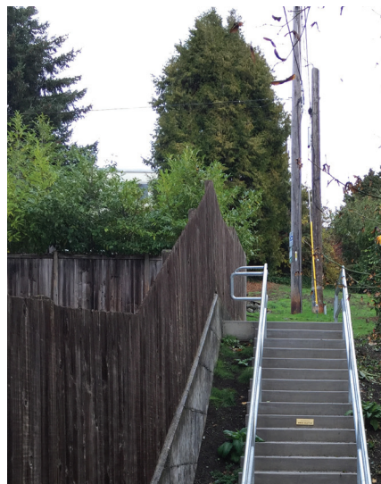
Stairway shown on right as inspected before replacement
