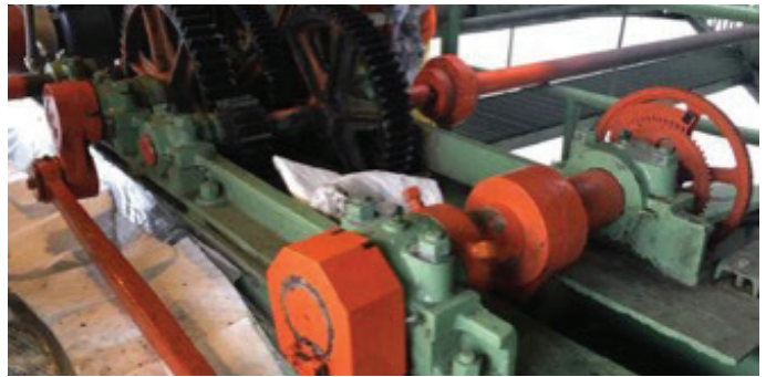
Ballard Bridge centerlock gears and lateral transfer shaft undergoing repairs
