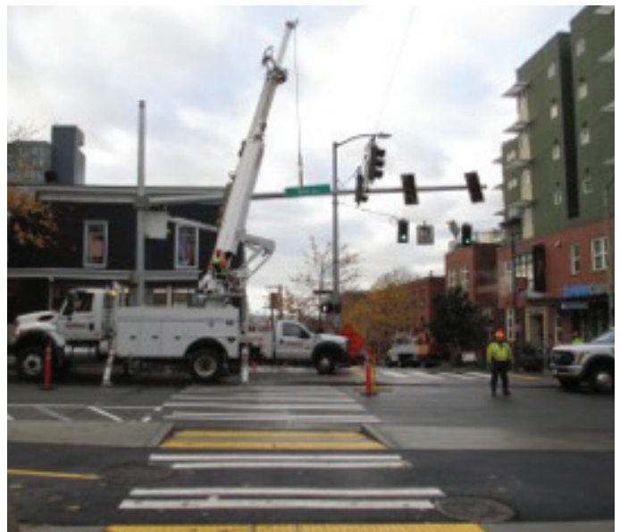
RIGHT: Installation of new signal at 2nd Ave and Bell St
