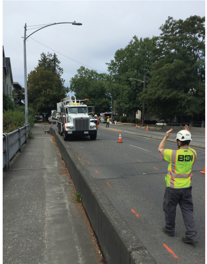
Live Load Rating at Admiral Way Bridge
