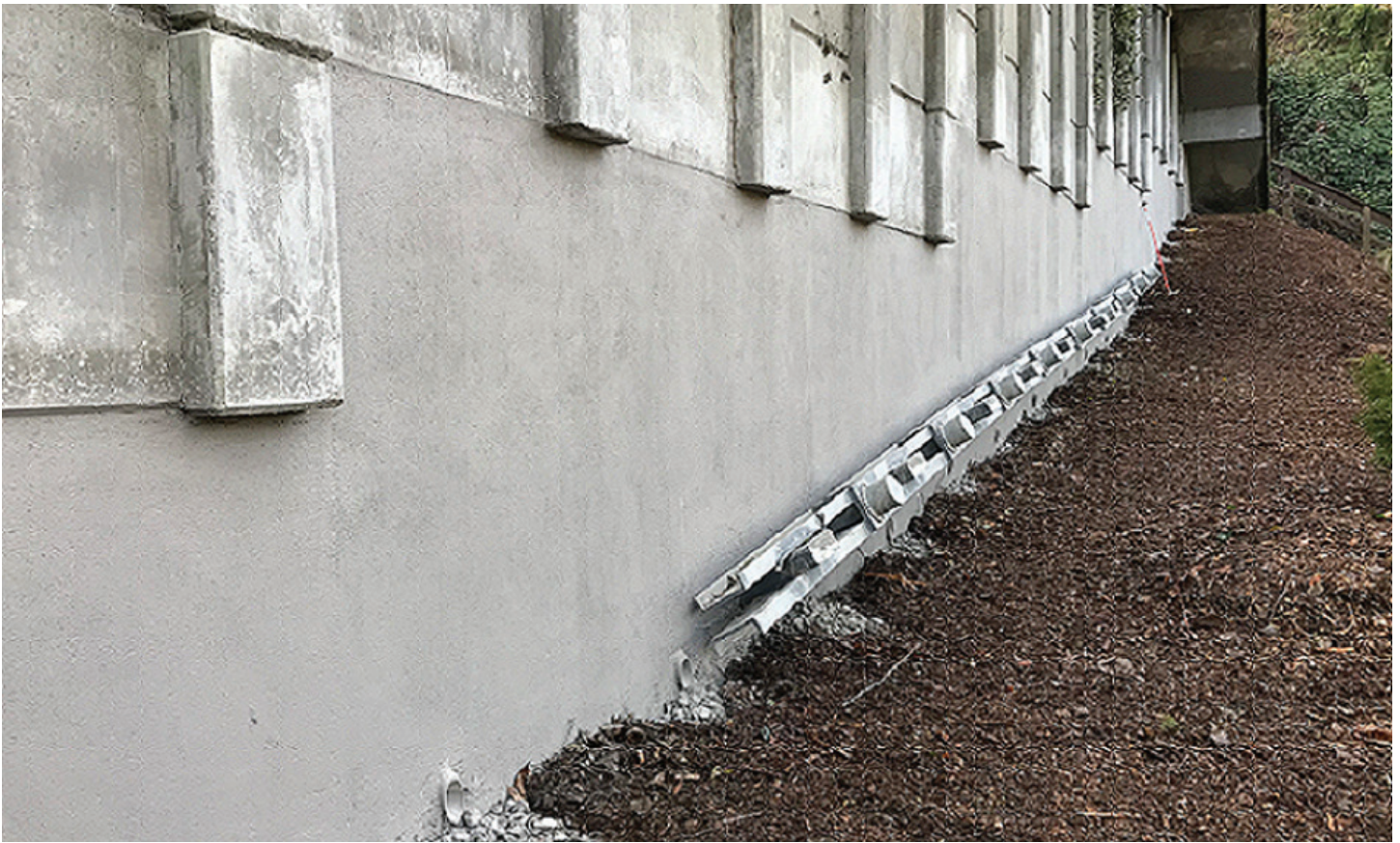
Retaining Wall at NE 98th and 20th Ave NE
